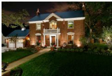
Here is the front elevation after.
